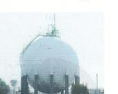
**Spherical Vessel.** Here the maximum stress occurs in any two perpendicular directions on an element of the vessel, Fig. 8–2a. From Eq. 8–3, we have
