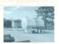
A cylindrical pressure vessel has an inner diameter of 1.2 m and a thickness of 12 mm. Determine the maximum internal pressure it can sustain so that neither its circumferential nor its longitudinal stress component exceeds 140 MPa. Under the same conditions, what is the maximum internal pressure that a similar-size spherical vessel can sustain?
